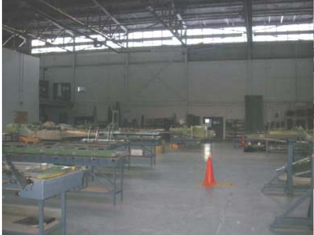
120-foot clear span assembly area, looking east.
