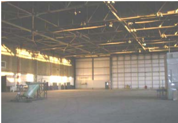
145-foot clear span – spare space, looking south. Clear height is 30 feet.
